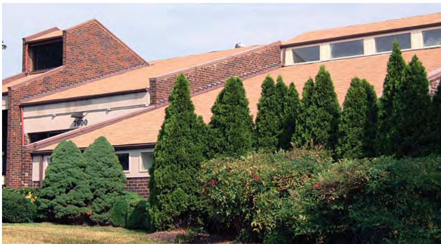
Greenbriar Community Building
